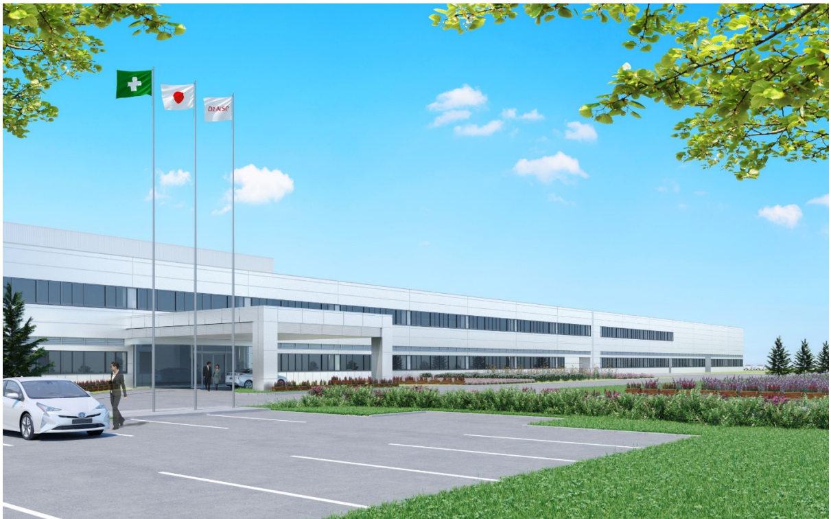
Completion image of DENSO Hokkaido Corporation after plant expansion
